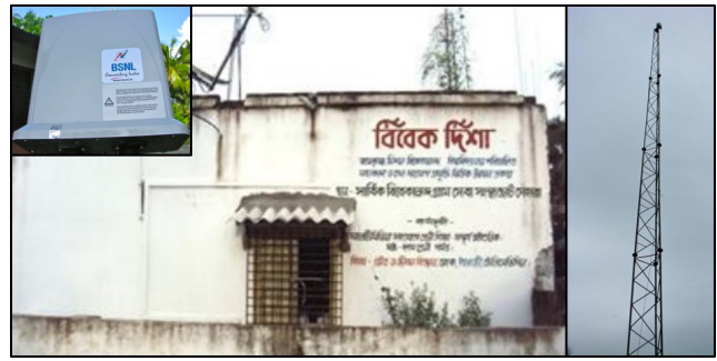
Fig. 4. A Vivekdisha's education and healthcare center equipped with our WiMAX-based last-mile telecommunication solution. Figure on the right shows the mast used to host the WiMAX CPE and figure in inset shows the WiMAX CPE that connects to the base station [23].
